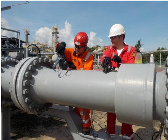
TOTAL E&P Brunei - SRUT on Monolithic Isolation Joint
