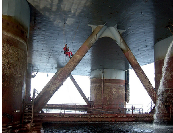
TOTAL E&P Congo – Complete Rig Inspection
