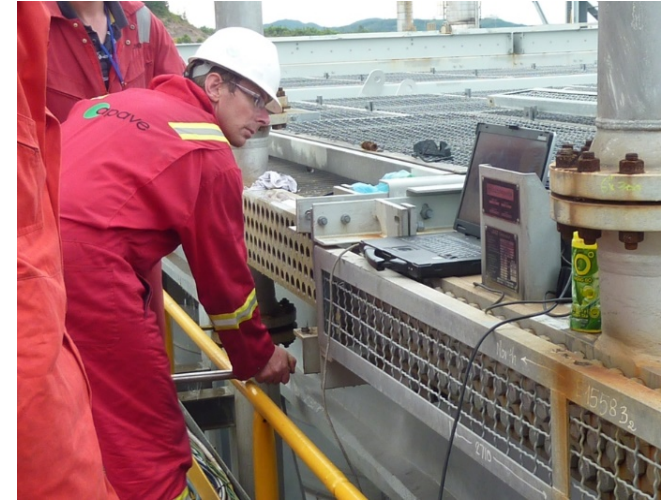
BSR, Vietnam - Tube inspection on Air Fin Cooler
