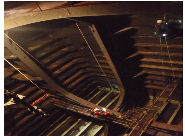
ExxonMobil, EG – Tank Integrity survey FPU ZP
