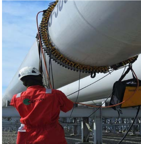
TEPB, Brunei - LRUT inspection on 42" Slug Catcher
