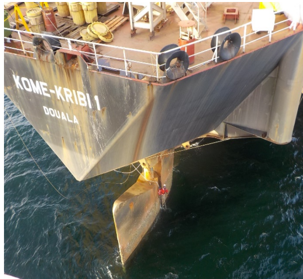
COTCO ExxonMobil, Cameroon – FSO Kome Kribi 1 Coating Maintenance
