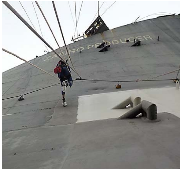
MEGI ExxonMobil, EG – FPU ZP Coating Maintenance
