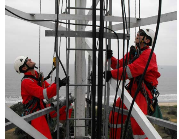
HESS EG, Bata Telecommunication Mast Structural/Corrosion Survey
