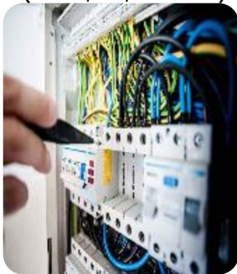
Inspection of Electrical Installations (ATEX, CP, DCVG...)
