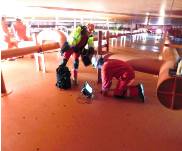
ENL, Russia - PAUT corrosion detection on Crude Oil Storage Tank TAR Dekastri Export Terminal
