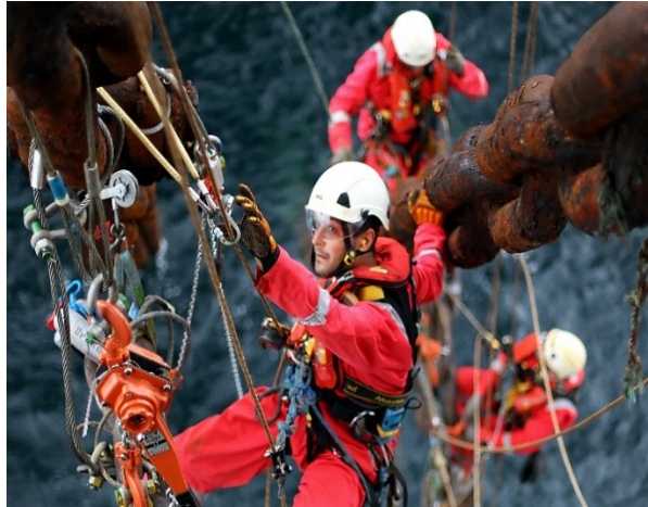
ExxonMobil, EG - Mooring chain's inspection according to ABS requirements
